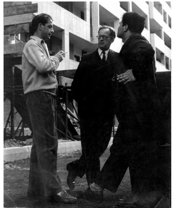
18 Denys Lasdun talking to Eduardo Paolozzi and Edwin Maxwell Fry on the building site of the Hallfield Estate, Paddington, c. 1955
